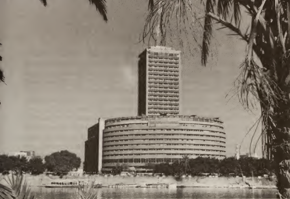
Government television building, Cairo Courtesy Embassy of Egypt, Washington
